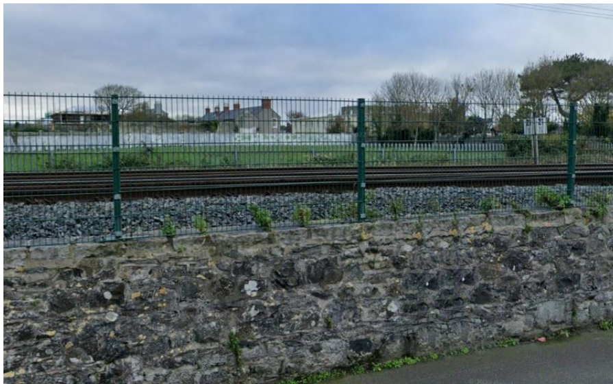
Plate 4-23 Paladin on masonry wall in Balbriggan (Google Maps)
