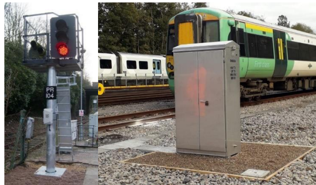
Plate 4-8 Example signal post & LOC cabinet (Source: Collis/ RSP)
