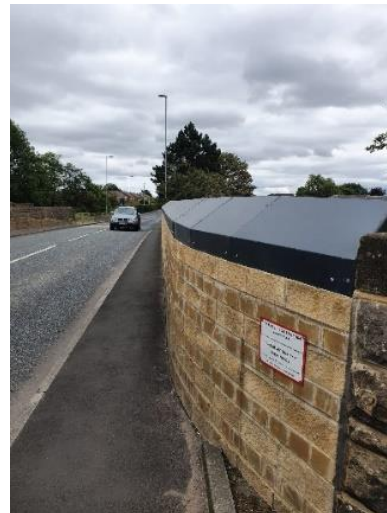
Plate 4-19 Typical bridge parapet wall height extenders
