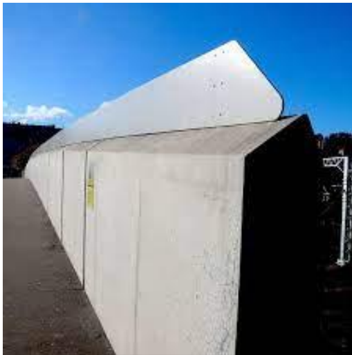
Plate 4-19 Typical bridge parapet wall height extenders
