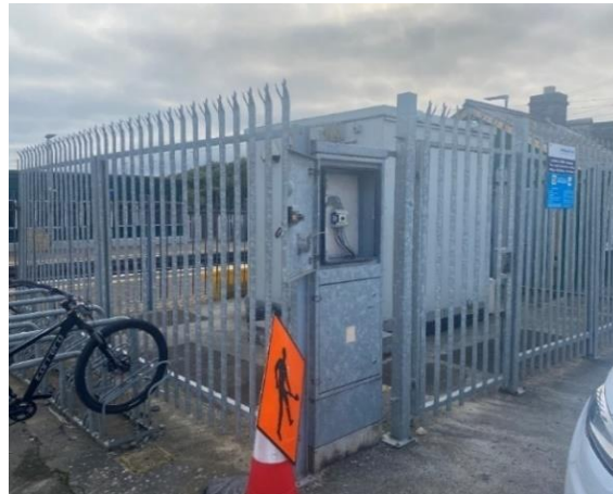
Plate 4-7 ESB LV supply point at Gormanston for TER (IE)
