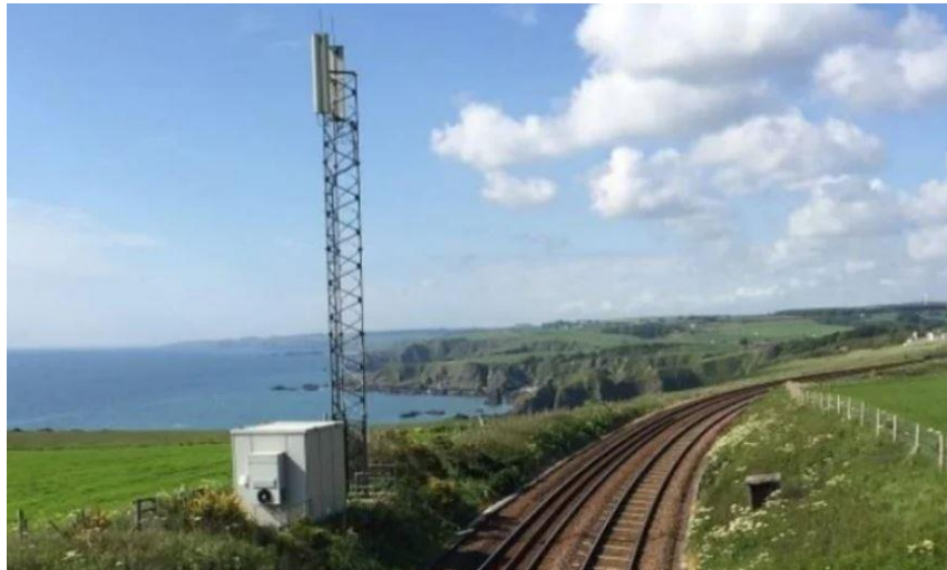
Plate 4-12 Example GSM Radio mast transceiver station
