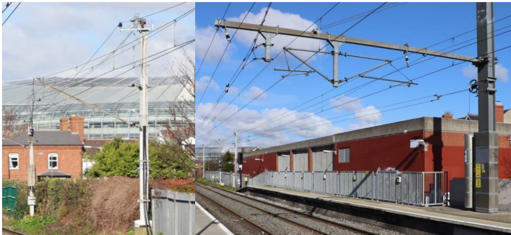
Plate 4-1 Example single & two-track cantilevers (Arup)
