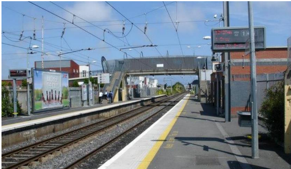
Plate 4-2 Example Headspan (DART)
