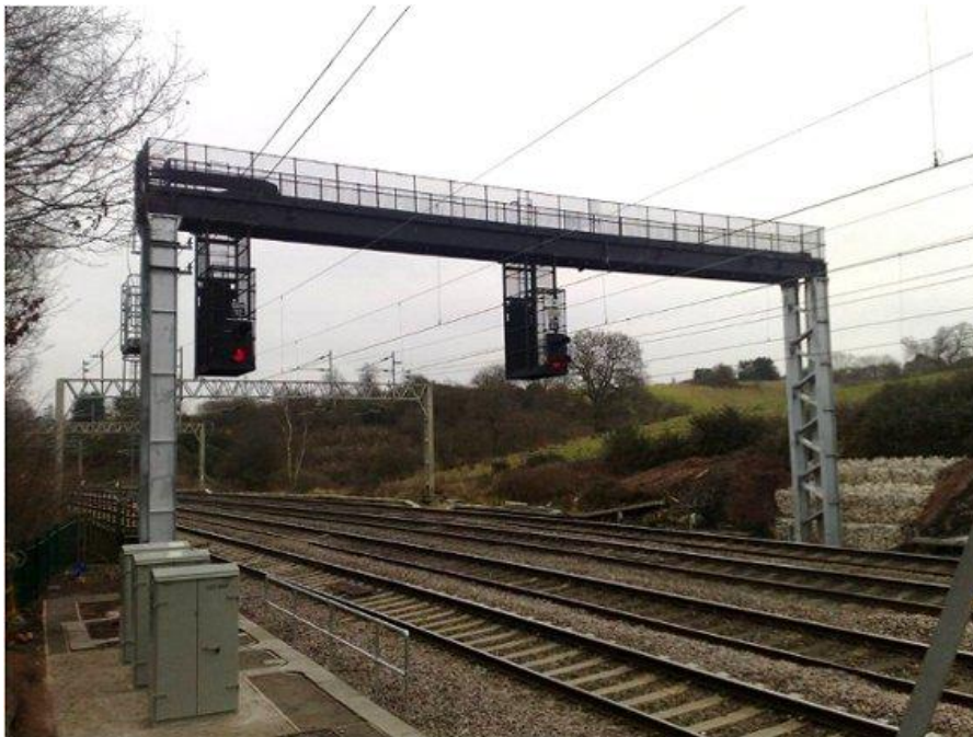
Plate 4-10 Example portal gantry (Source: Fli Structures)
