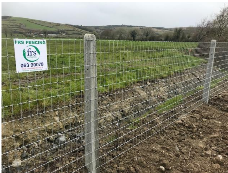
Plate 4-21 Concrete post and wire with stock proof mesh
