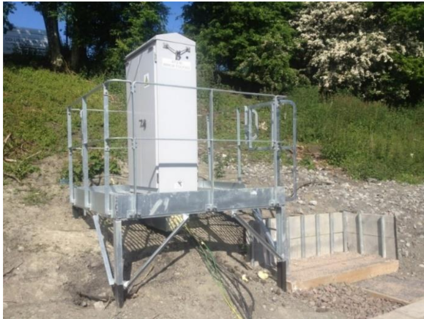
Plate 4-11 Example signal LOC installed on a platform (Source: Collis)
