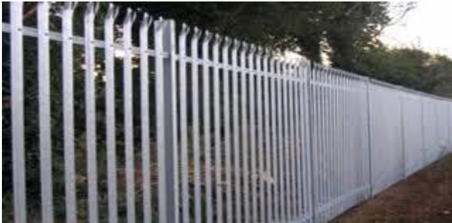
Plate 4-20 Palisade fencing
