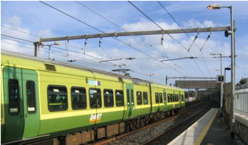
Plate 4-3 Example portal frame (DART)
